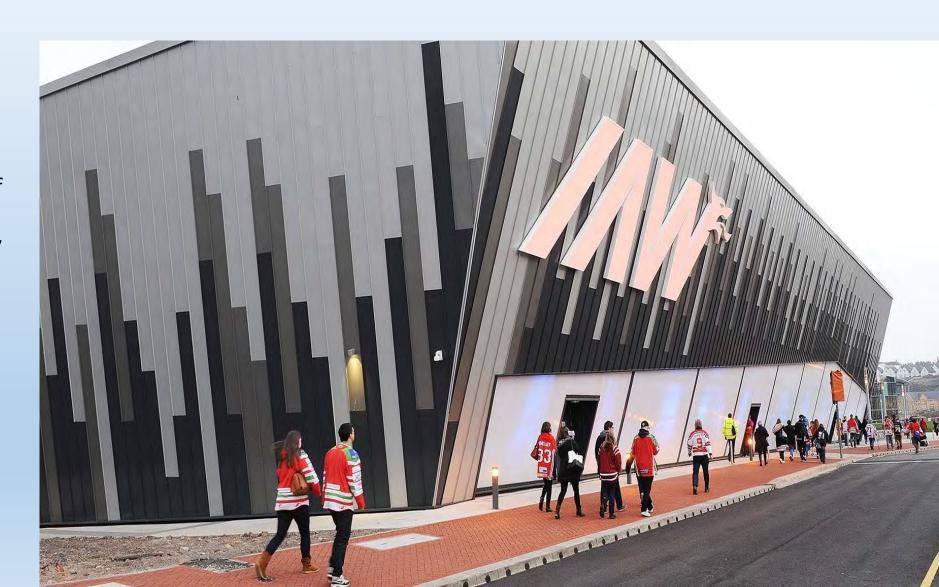
It is a striking building of steel frame construction with dark to silver metal cladding with a gently raked roofs with angled walls that give the building a distinct character which extends to approximately 8,336m<sup>2</sup> (89,728 ft<sup>2</sup>) Gross Internal Area (including areas of plant and services).
